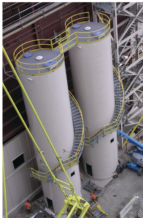
(2) Factory-welded and buyer supplied equipment installed in Winchester, TN and shipped to Colorado, storing powder activated carbon.
