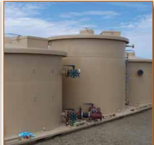
**PetroTec Welded** – Factory welded and coated with our proprietary coating system to ensure maximum corrosion resistance and long tank life.
