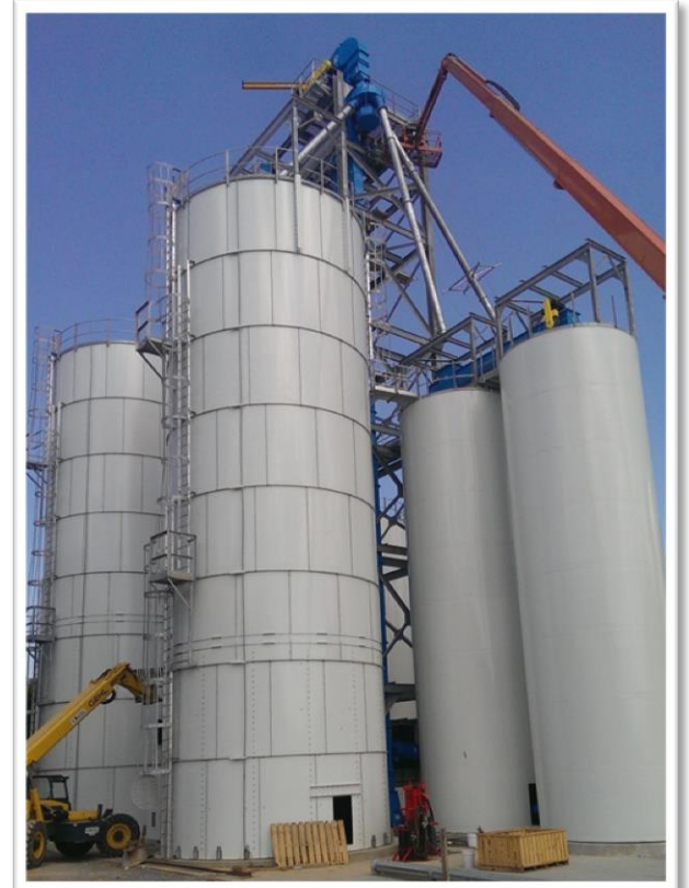
CST Storage tanks being installed at the Jack Daniel's facility
