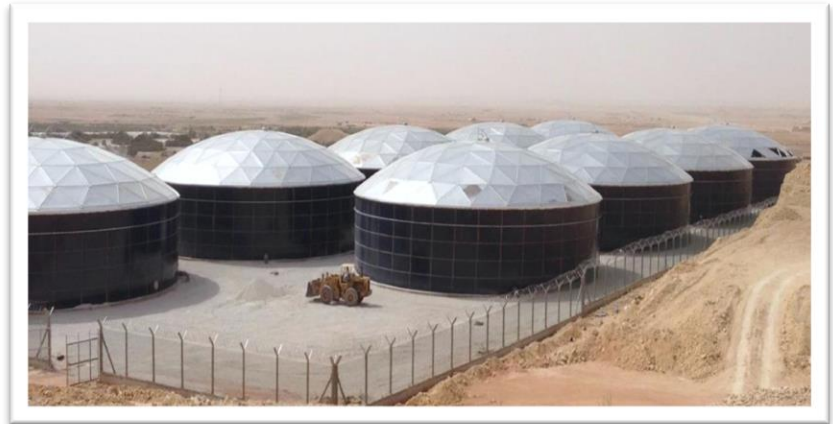
Tanks identical in size storing 5,000 cubic meters with dimensions of 31.5m diameter and 6.9m height.
