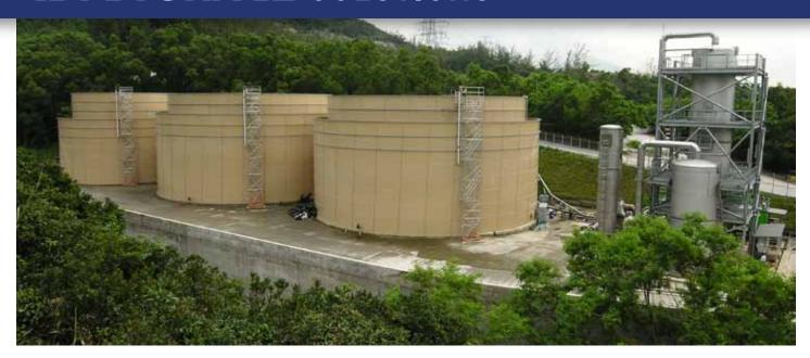
of safety in mind, CST recommended the use of its TecStore tanks, which offered the same technologically advanced coatings for abrasion and corrosion resistance, but utilized a jack system in place of a scaffolding system for installation.
