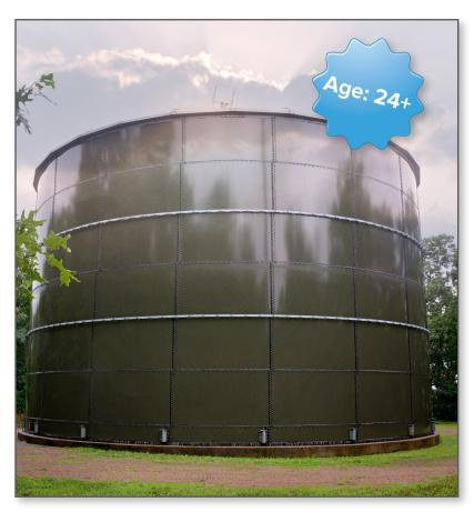
glass fused to steel. A municipal water provider in South Dakota estimates that maintenance for a glass-fused to steel tank over a 60-year span would cost \$266,000 compared for \$906,000 for a painted welded tank.
