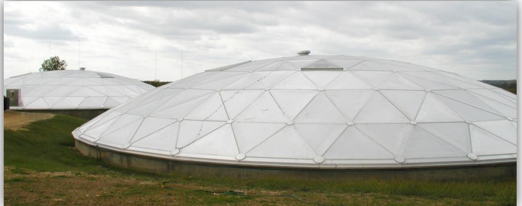
Gracon reviewed proposals from three manufacturers. While two presented similar roof designs, CST Covers recommended fully interlocking panels, which are easier to fabricate on site. The CST dome roofs require significantly less time and labor for installation and provide a long-lasting, durable and extremely low-maintenance solution.
