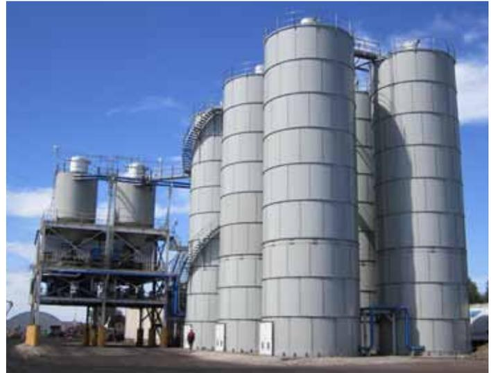
CST Storage (formerly Columbian TecTank), Norit America's storage partner, was given the task of building eight tanks – six steel bolted panel tanks which would store the PAC upon arrival from Texas by rail, and two factory welded tanks with component in tank (CIT) equipment preinstalled by CST Storage to load the PAC into trucks for delivery.
