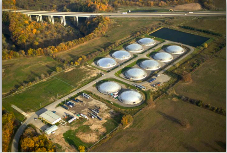
Greatario Engineered Storage Systems: An overview of the aluminum covers for wastewater treatment at Halton Region, Ontario, Canada.
