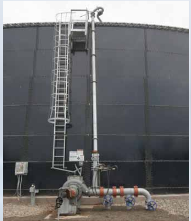
Slurrystore 2400 Pump with Deluxe Over-the-Top Agitation Nozzle
