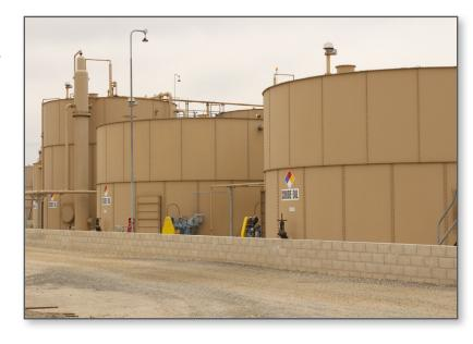
agricultural markets. The project's scope was significant—replace the existing tanks, consolidate the pipeline and reduce the tank farm's footprint from 1.6 acres to just a half acre.
