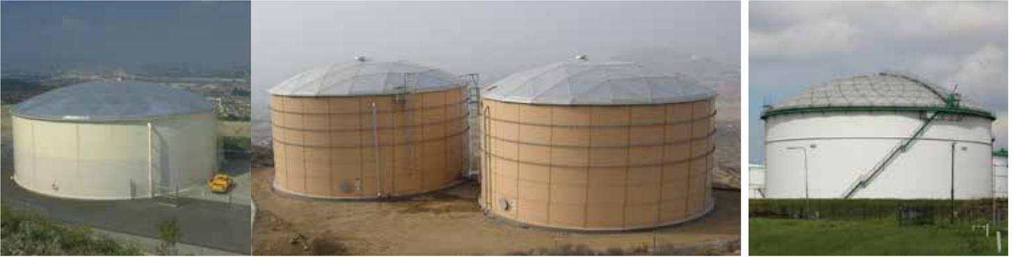
CST Covers is the first choice for thousands of petrochemical applications worldwide. Always featuring all-aluminum construction, CST Covers products are lightweight, corrosion-resistant and maintenance free, which translates to longer life and lower costs. They don't rust like steel, they don't degrade with ultraviolet light like fiberglass, and they don't spall like concrete. Their strength and versatility are unmatched.
