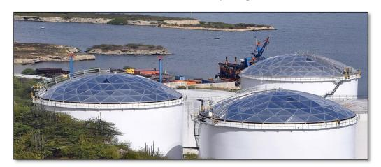
In early 2012, a general contractor was awarded a project by a local fuel and gas distribution company in Willemstad, Curação to design and construct three API 650 tanks for the purpose of storing liquid fuel oil. Each tank was to be 36.6 m (120 ft) in diameter and 17.7 m (58 ft) in height, with a nominal storage capacity of 17.000m3 each. The three new tanks would be integrated with the other tanks and would store fuel oil and marine fuel.
