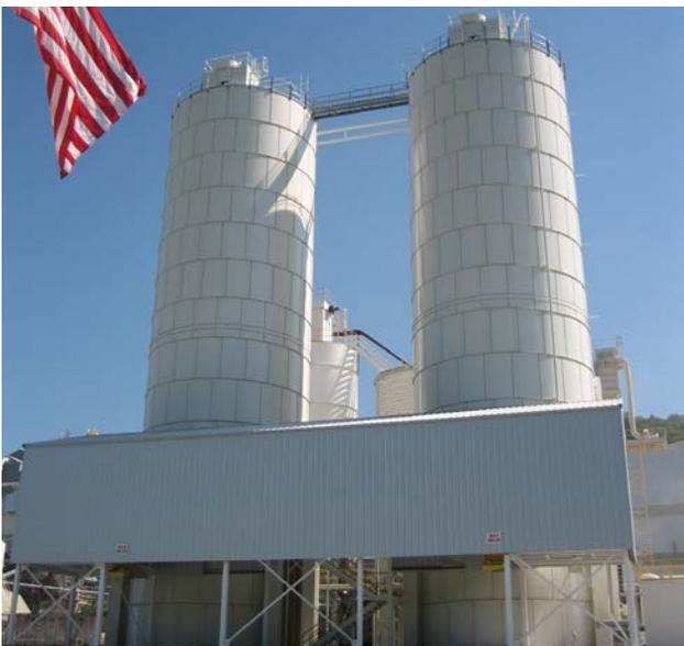
(2) 32' x 112' with dual capability to loadout both truck and rail.
