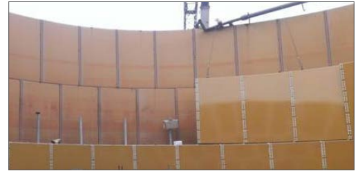
>> Corroded Staves Replacement
