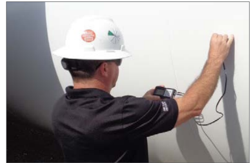
>> Ultrasonic Thickness Testing - Carbon
