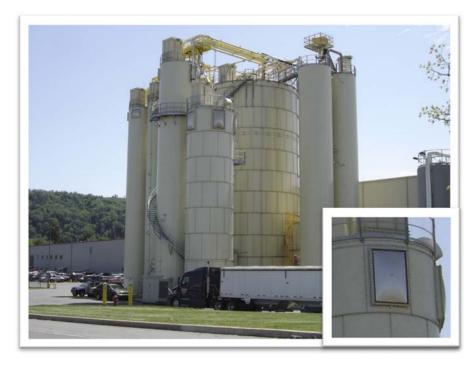
on how to prevent silo damage or equipment failure from future explosions. Sweet suggested "explosion relief vents," which are a series of vents near the top of the tank's sidewall that allow the combustible gases to escape and lower the pressure inside the silo.
