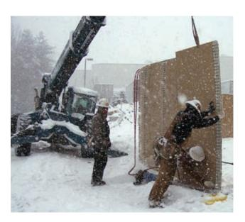
Chime panel tank assembly typically involves scaffolding methods. Special scaffolding mounts and assembly ladders increase construction efficiencies and safety.
