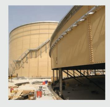
Flat panel tanks are typically assembled from the top down by using a hydraulic actuated, synchronized jacking system that is third party proof load tested and PE stamped.
