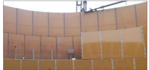
>> Corroded Staves Replacement
