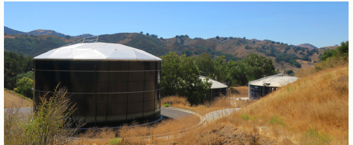
↑ Ground Storage Tank
